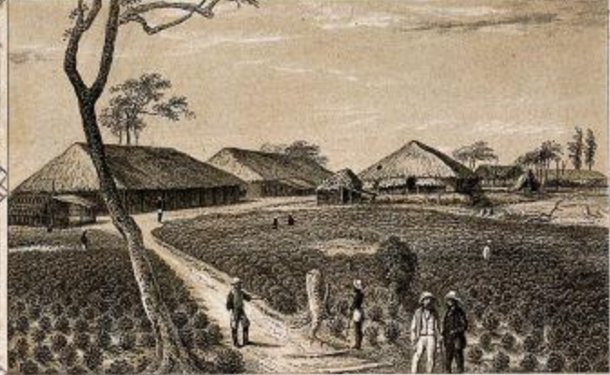
NEW STATION, ROSEKANDY COOLIE LINES ASSAM.
